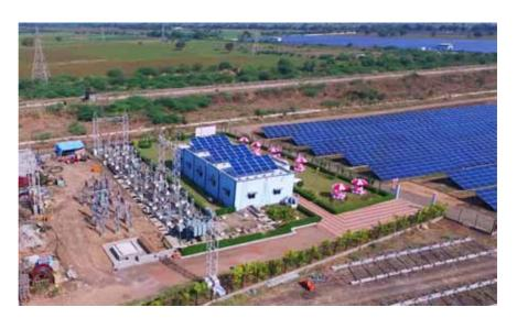
had capacity to transfer 30 mw. Post changes in infrastructure, the company increased evacuation capacity to 70 mw. GETCO approved the same in July 2019. In fact, our transmission infrastructure, equipped with double circuit of 'Panther' conductors, can enable transmission up to 100 mw.
